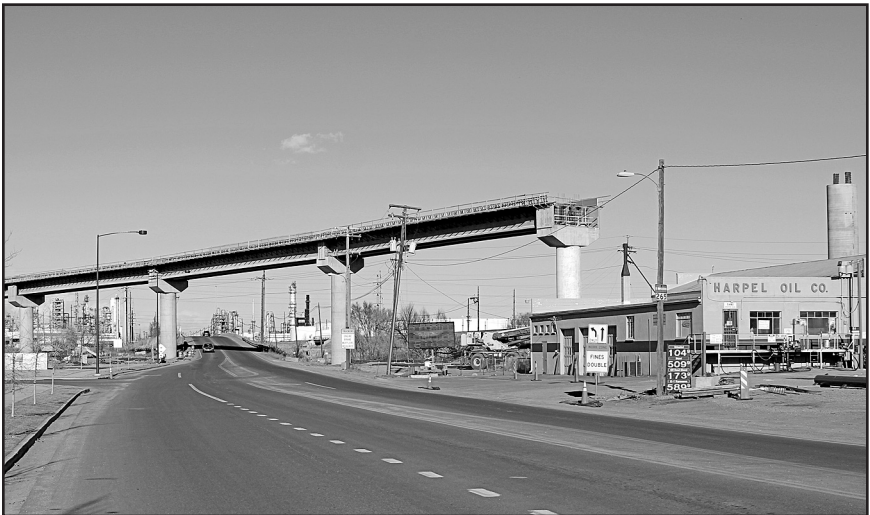
Bridge construction on a new RTD commuter line on February 20, 2016, seen here crossing Brighton Boulevard in the 5500 block in northeast Denver. This structure will also carry the RTD track over the BNSF Brush Subdivision and the U.P. Belt Line. – Photo © 2016 Dave Schaaf.
